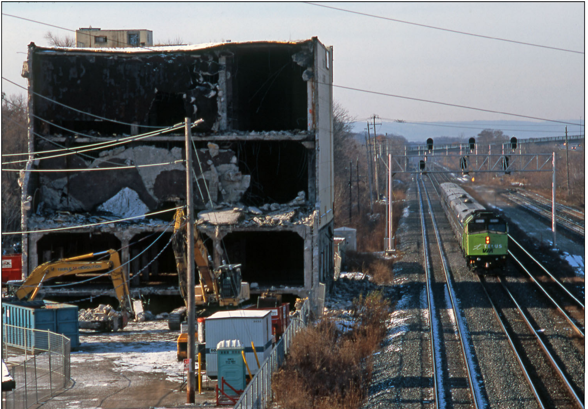
Aldershot Cold Storage R.I.P. A decades old landmark in the Burlington area has always been the Aldershot Cold Storage facility West of Waterdown road. Built in the 1930s for area farmers requiring refrigerated storage of fruit and vegetables, the end is now here as a crew from Triple M Demolition chews away at the reinforced concrete structure. While in operation in the 1970s, an active siding existed where David R Howard the new Oakville Sub 3rd mainline is now located. That's VIA #70 with the Telus 2010 Olympics unit passing by. A Morgan's Caboose Production
