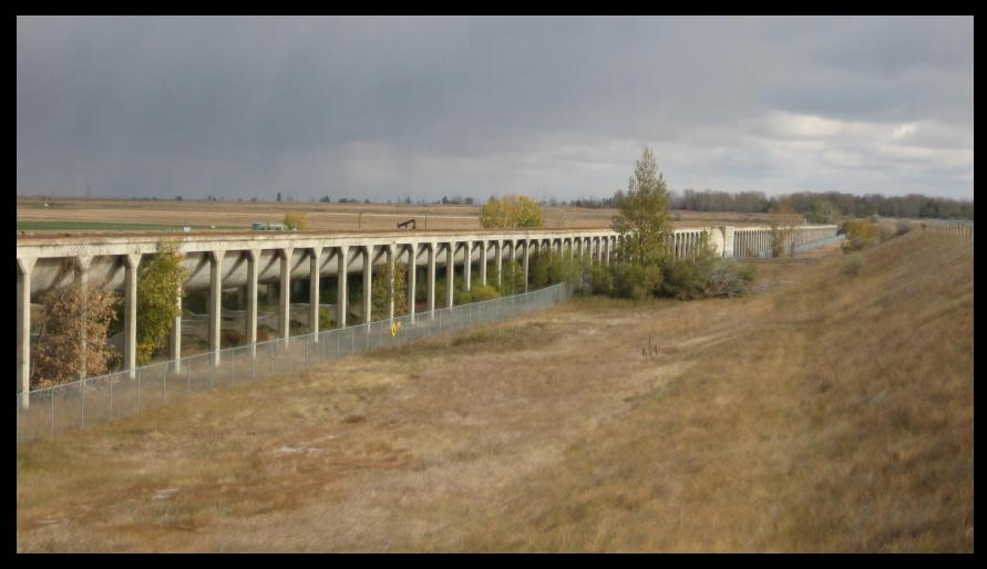
The eastern portion of the Brooks Aqueduct on 10 Oct 2009; the irrigation water flowed in the half-round steel lined concrete flume supported by the concrete pillars. To the right of the large tree the inverted portion of the aqueduct can be seen, where a concrete pipe carried the 640 cubic feet per second of water under the CPR main line. The aqueduct is a National Historic Site (since 1983).
