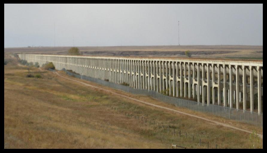
The CPR built the Brooks Aqueduct (west side seen here on 10 Oct 2009) between 1911 and 1914 to carry irrigation water from the Bassano Dam across this valley east of Brooks to the Millicent, Tilley & Patricia areas. The aqueduct is 2 miles long and 61 feet high. It was taken over by the Eastern Irrigation District in 1935; it was replaced in 1979 by a raised earthen embankment with a canal.
